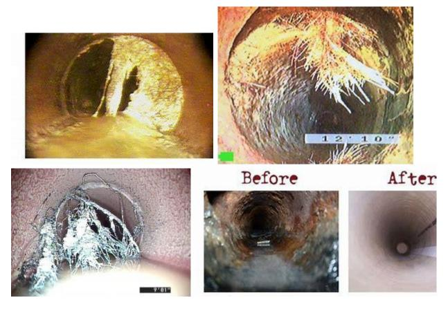
Cured in Place Pipe provides a new liner that stops root infestation and provided additional structure to the pipe.
